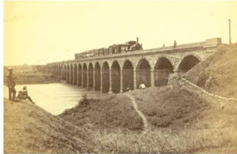
First Railway Bridge linking Bombay with Thane, 1854
